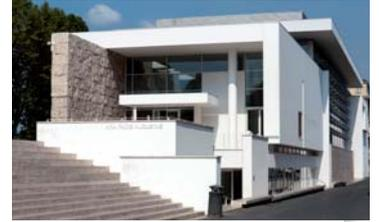
It is a long, single-storey glazed loggia and replaces the previous enclosure which was in ruins. The new structure has all the features of Meier's design, in particular his expansive use of glass. The glass loggia stands above a shallow podium and provides a transparent wall between the river Tiber and the circular perimeter of the mausoleum of Augustus, built about 28 BC. The building consists of an asymmetrical entry hall with seven reinforced concrete columns finished with white waxed marble
